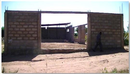
Church building in construction in Usagala mission area.
