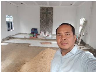
Looking from the inside before completion.
